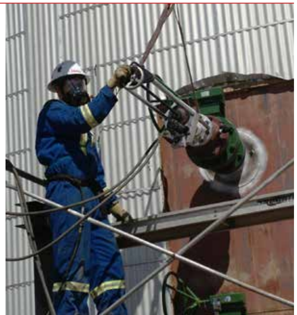
Standard Hot Tap on an Oil Refinery Storage Tank
