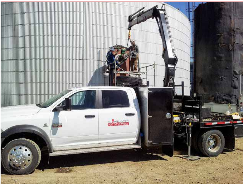
Standard Hot Tap on an Oil Refinery Storage Tank
