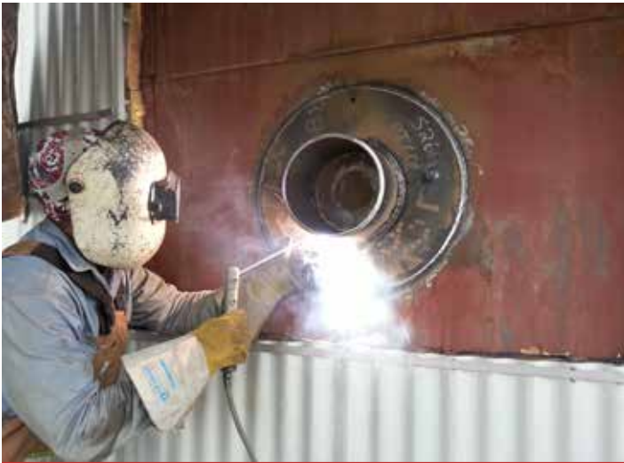
Standard Hot Tap on an Oil Refinery Storage Tank
