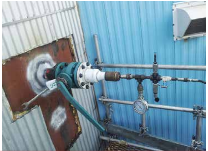
Standard Hot Tap on an Oil Refinery Storage Tank
